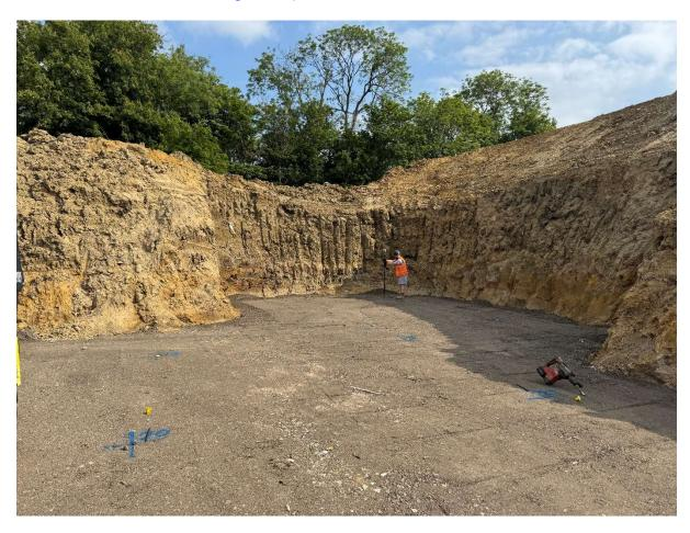
The image shows a significant excavation with exposed earth banks and a surveyor working in a dangerous location at the foot of the excavation. There is also a type of drill lying on the ground which could present a trip hazard. Several potential safety implications related to UK construction law and regulations are evident.
